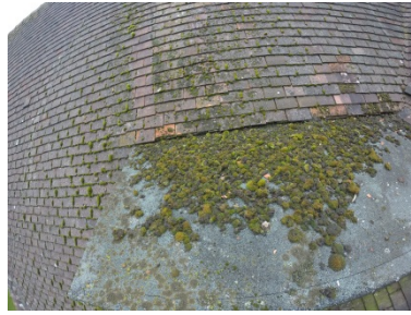
Spalled roof tiles
