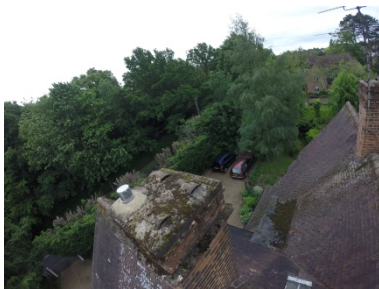
Loose and defective flaunching
