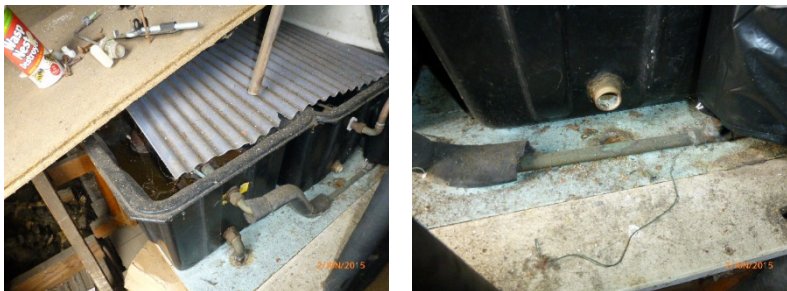
Expansion tanks covered in plastic Pipes are not fully insulated
