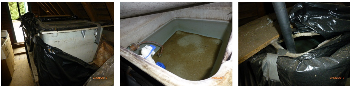
Cold water storage tanks are poorly sealed and the water is contaminated
