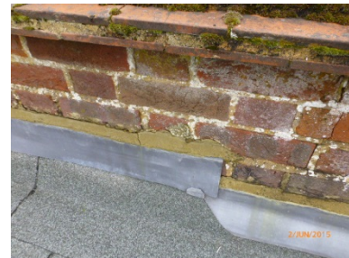
Loose and defective pointing to the rear flat roof flashings
