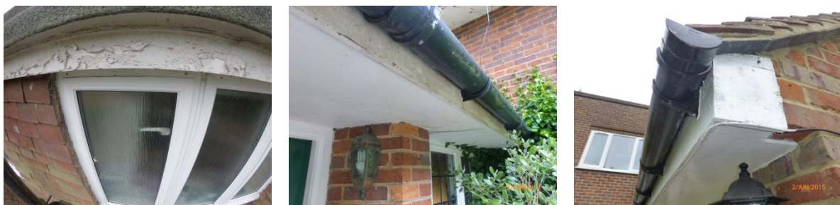
Decoration to the soffit and fascia boards is in a poor state of repair
