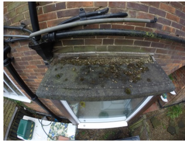
Side bay roof is worn
