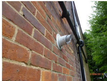
Fan assisted flue
