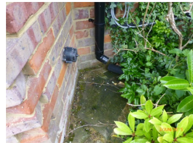
Rainwater pipe not connect to soakaway
