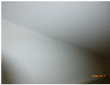
Cracking to the ceiling line
