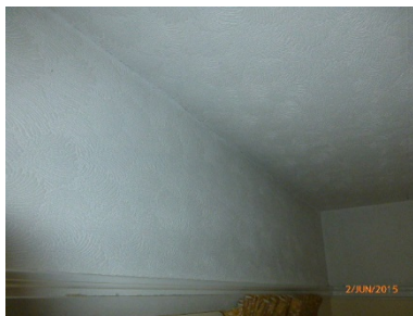
Cracks to the ceiling line
