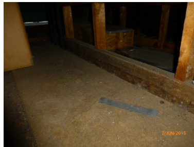
Rear loft is fully boarded and not adequately insulated
