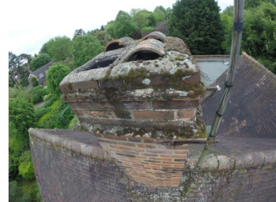
Loose and defective pointing
