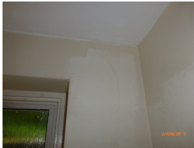
Cracks to the walls and the ceiling
