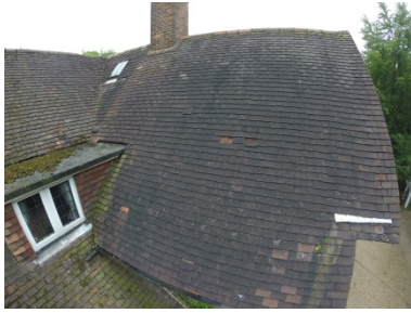
Missing/slipped/broken roof tiles
