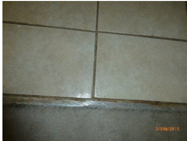
Floor tiles are loose and the joints are cracked
