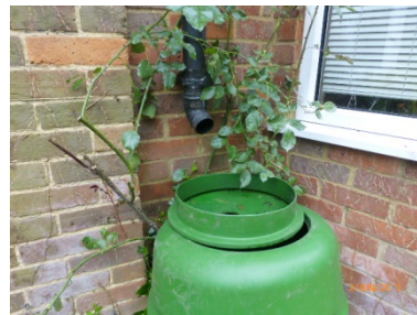
Pipe cut short of water butt
