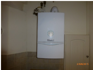
Wall mounted boiler
