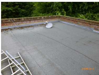
Parapet walls are too low
