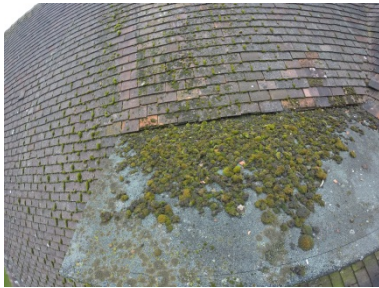
Front bay roof is worn
