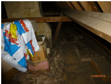
Front loft fully insulated
