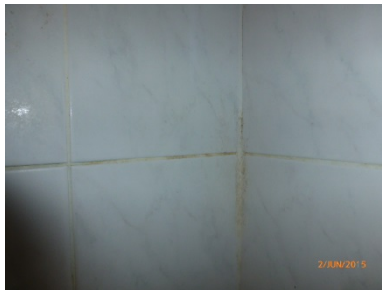
Sealant to the abutments is poorly finished
