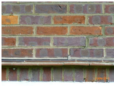
Deflection to the brickwork above the rear facing window
