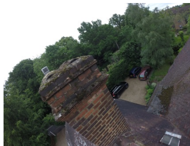
Poorly capped flues
