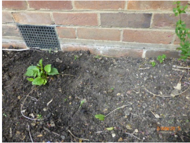
Ground levels to the front side and rear are finished too high compared to the DPC
