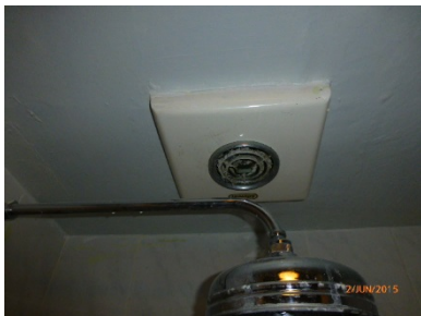
Ceiling mounted extractor
