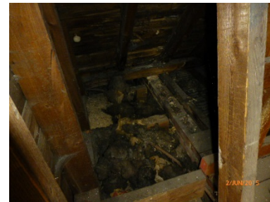
Rear loft is fully boarded and not adequately insulated
