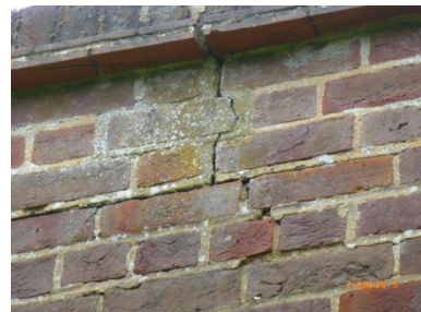
Crack to the side rear parapet wall
