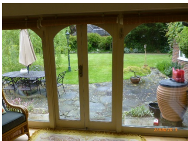
Glass to glazing panels is not correctly etched to confirm compliance
