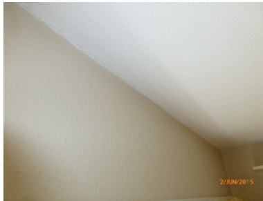
Cracks to the ceiling line
