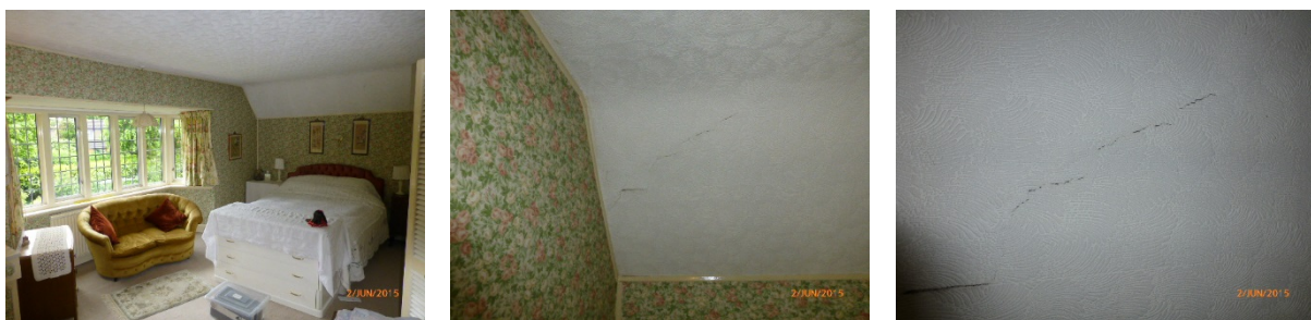
Crack to the skirting
