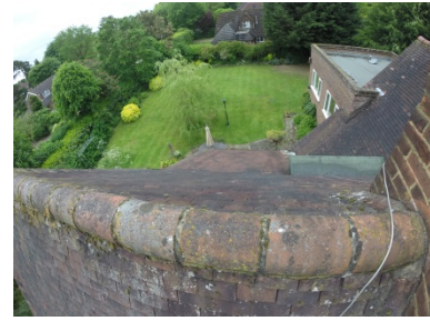
Loose and defective ridge mortar
