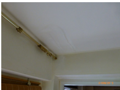
Water mark to the ceiling and blistering to the wall paint
