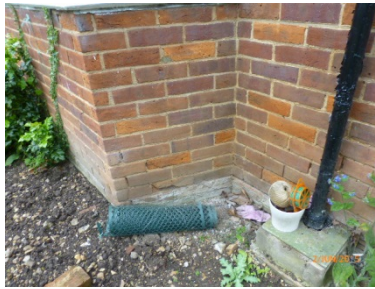
Loose pointing and spalled brickwork to the front and left side
