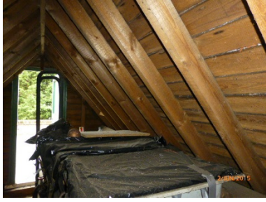
Roof is well constructed braced and supported
