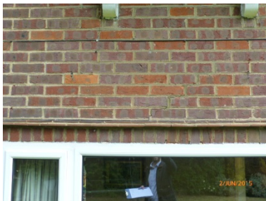
Deflection to the brickwork above the rear facing window
