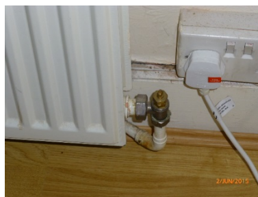
Not all radiators are fitted with TRV's
