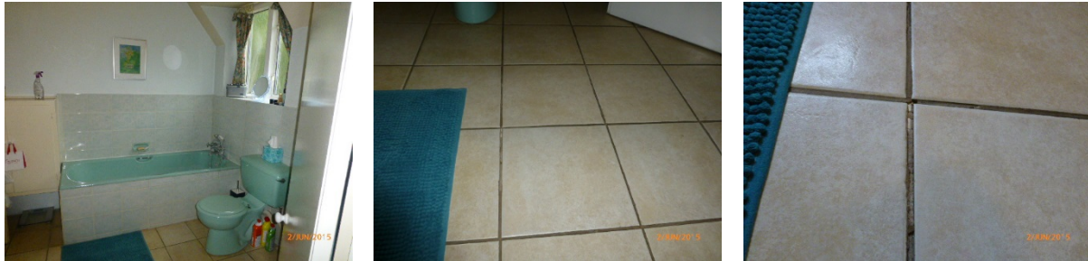
Floor tiles are loose and the joints are cracked
