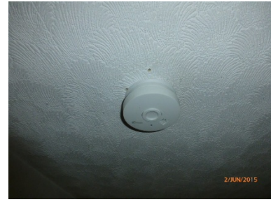
Battery powered smoke detection
