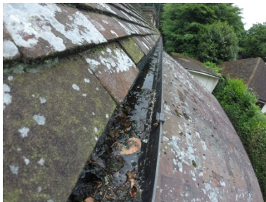
Gutters contain moss and debris
