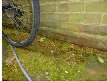
Ground levels to the front side and rear are finished too high compared to the DPC
