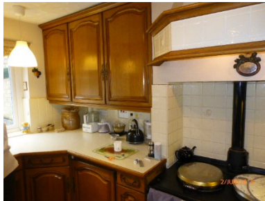
Extraction is not externally ducted
