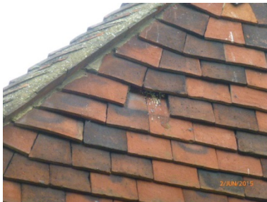
Missing hanging tiles to the various elevations
