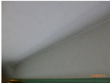
Cracks to the ceiling line
