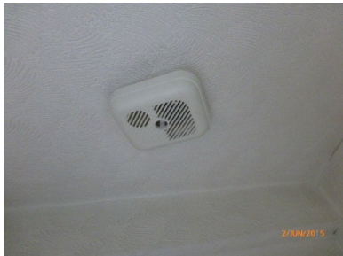
Battery powered smoke detection
