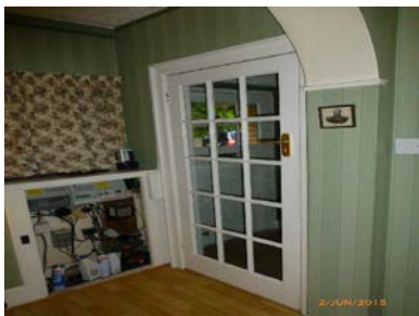
Glass in a critical location
