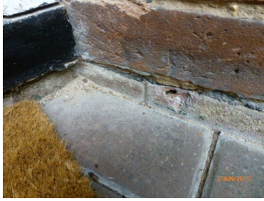
Bitumen DPC to the front and sides
