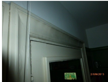
Staining to the door surround
