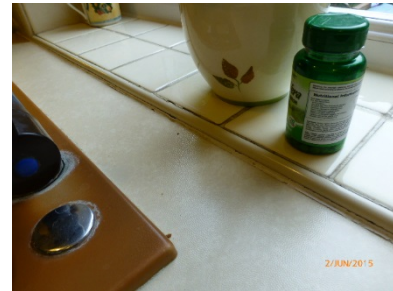
Sealant to the worktops is poor
