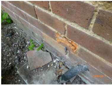
Loose pointing and spalled brickwork to the front and left side
