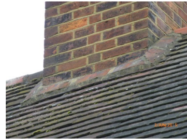
Abutments are poorly sealed
