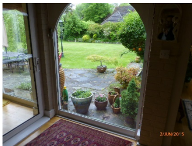
Glass to glazing panels is not correctly etched to confirm compliance
