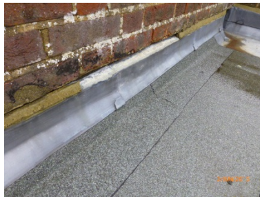
Loose and defective pointing to the rear flat roof flashings
