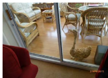
Glass to the doors and windows is in a critical location
