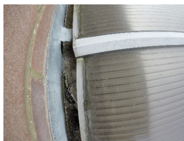
Narrow box gutter to both sides of the conservatory
