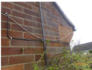
Poorly fitted cables to the front left and the rear
