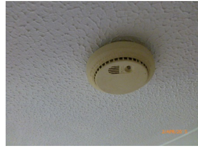
Battery powered smoke detection
