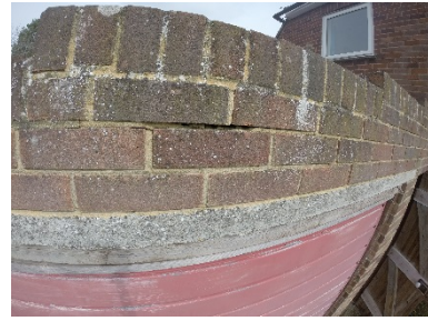
Garage parapet is loose and defective
