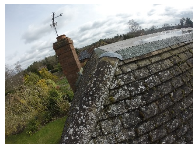
Poorly fitted lead to rear hips
