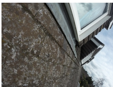
Lead aprons have been poorly fitted and are ridging
