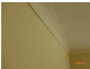
Cracks to the coving joints
