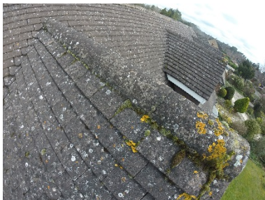
Ridge and hip mortar has cracked
