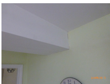
Cracking to the ceiling line around the drop down beam
