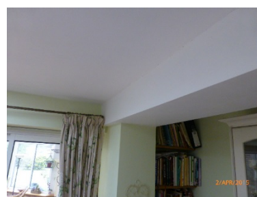
Cracking to the ceiling line around the drop down beam
