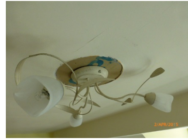
Poor finish around the light
