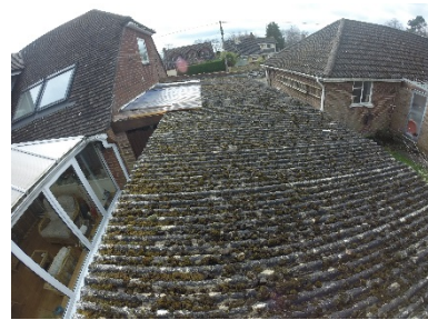
Potential ACM to garage roof
