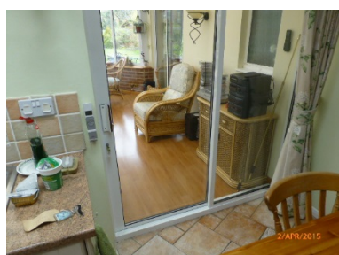
Glass to both doors is in a critical location
