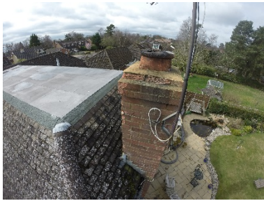
Rear chimney services the lounge Spalled bricks & cracked flaunching Open flue
