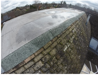
Apron has been laid in felt
