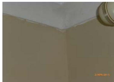
Cracks to the coving joints
