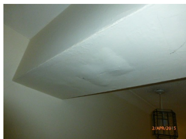
Damage to beam boxing
