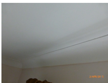
Cracks to the coving joints
