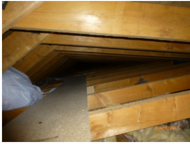
Roof is constructed in untreated timber
