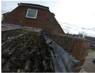
Poor flashing to garage parapet wall
