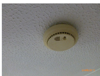
Battery powered smoke detection
