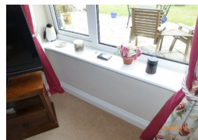
Glass to the doors and windows is in a critical location
