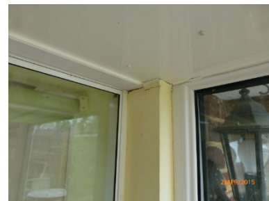
Cracks to the tops of the walls and around the window/door frames
