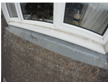
Lead aprons have been poorly fitted and are ridging
