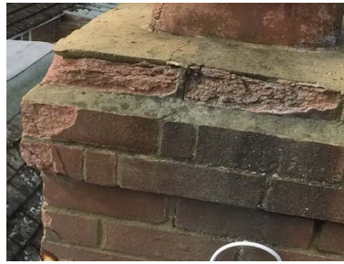
Rear chimney services the lounge Spalled bricks & cracked flaunching Open flue
