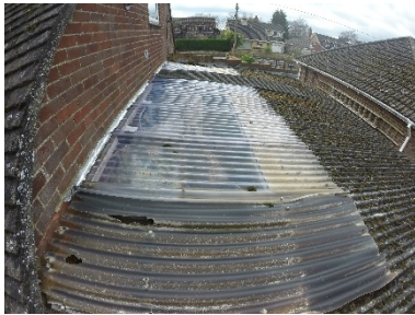
Poor flashing to garage roof
