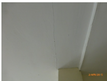
Cracks to the landing ceiling
