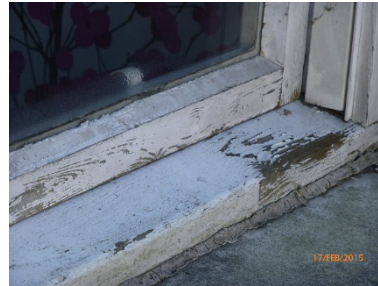
Window frames are in a poor state of repair particularly to the rear
