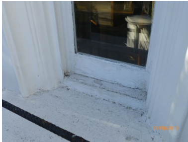
Window frames are in a poor state of repair particularly to the rear
