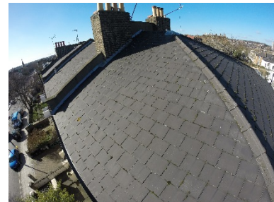
Front roof slope
