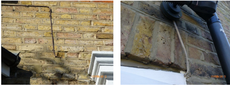
Poorly fitted cables to the front and rear
