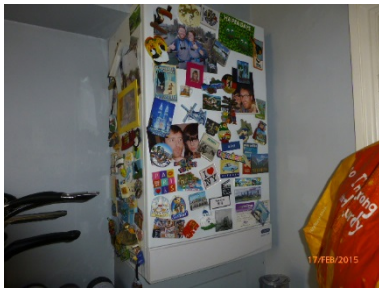
Wall mounted boiler
