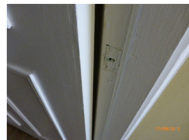
No smoke seals or intumescent seals fitted and closers removed
