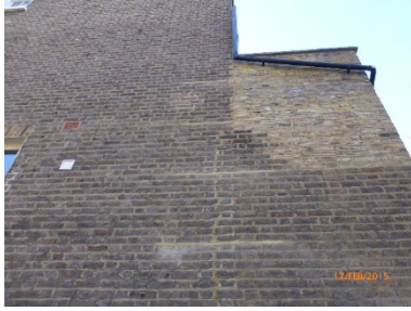
Evidence of structural repairs to the rear section of the side wall
