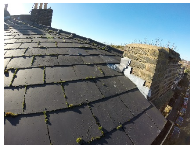
Side rear chimney
