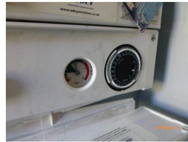
Built in controls
