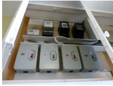
Main fuse and meter
