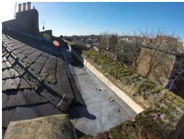
Copings to the rear parapet wall are poor
