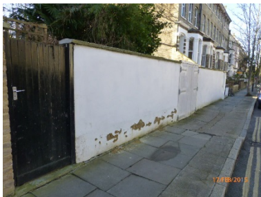
Saturation to the base of the render
