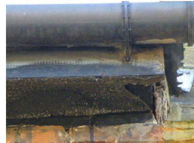
Soffit and fascia decoration is poor
