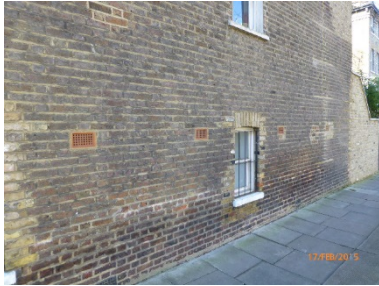
Pointing to the base of the side wall and the front stairs is loose and defective
