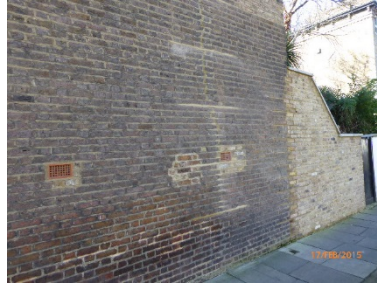
Evidence of structural repairs to the rear section of the side wall
