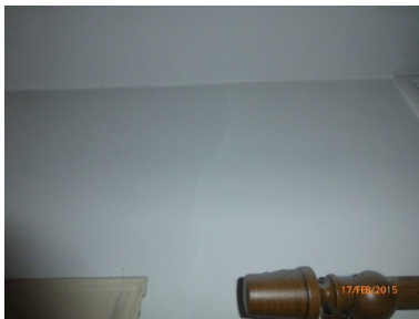
Crack to the rear external wall
