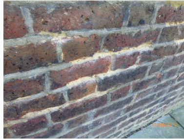
Pointing to the base of the side wall and the front stairs is loose and defective
