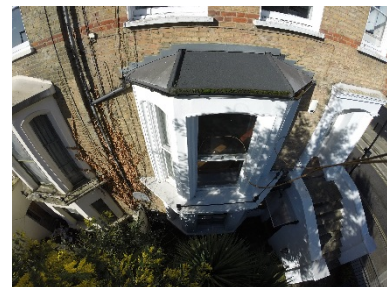
Poor repair to the front bay window
