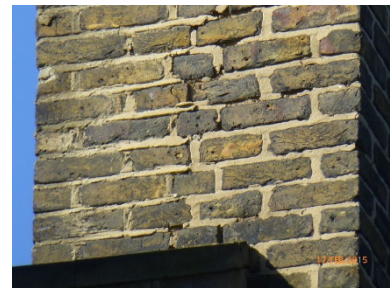
Loose and defective pointing
