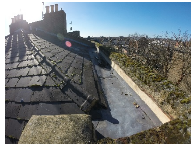
Rear roof slope
