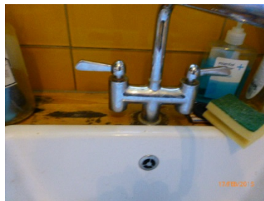
Tap is loose
