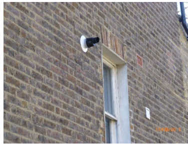
Fan assisted flue
