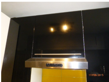
Extractor not externally ducted
