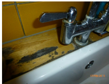
Water damage to the woodblock worktops around the sink
