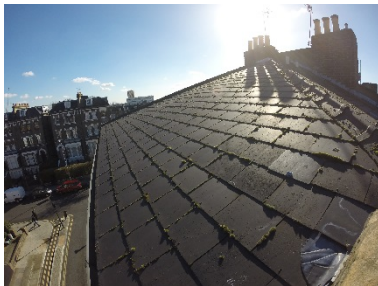
Side roof slope
