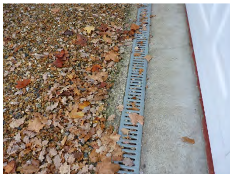
Rainwater gulley full of leaves and shingle
