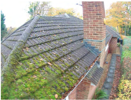
Heavy moss covering to the roof tiles
