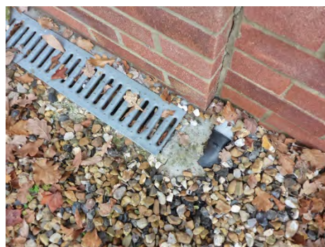
Rainwater pipe connected to gulley
