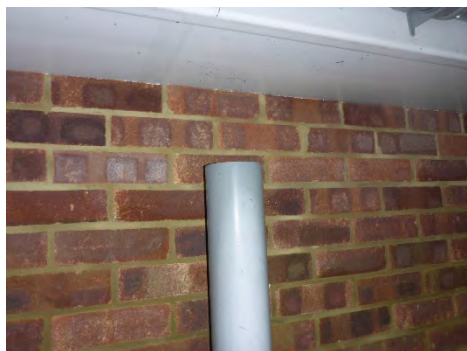
No cap to side vent pipe
