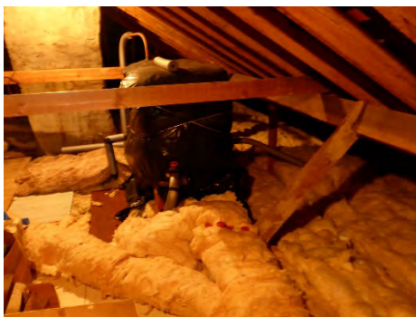
Insulation beneath the tank stand
