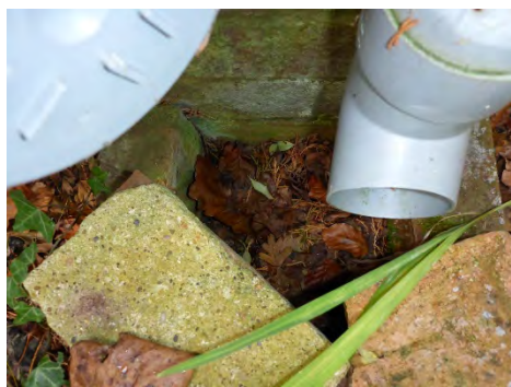
Blocked and open hoppers to the side and rear
