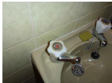
No sealant to the wash hand basin
