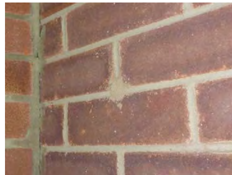
Evidence of retrospective cavity insulation having been injected
