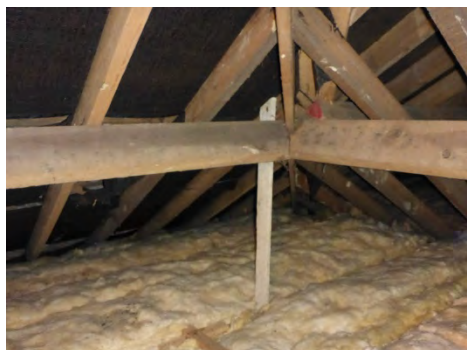
Hand cut roof is well braced and supported to the main building
