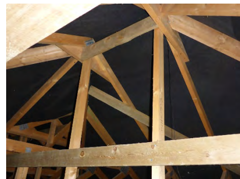
Trussed timber roof above extension
