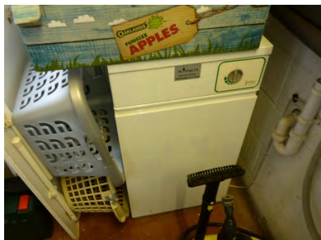
Floor standing oil fired boiler
