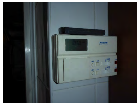
Boiler programmer
