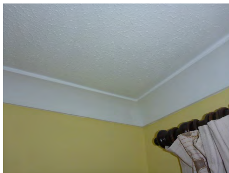
Cracks to the coving
