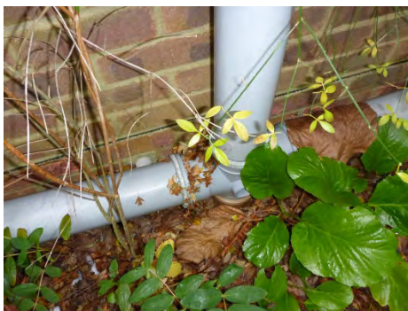
Inadequate rodding to the drainage
