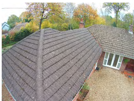
No visible means of ventilation to the roof timbers
