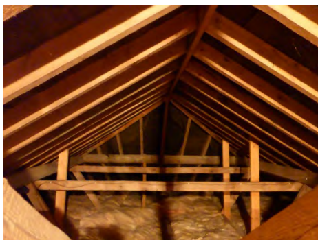
Hand cut roof is well braced and supported to the main building
