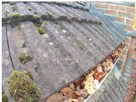
Gutters are full of leaves, moss and debris
