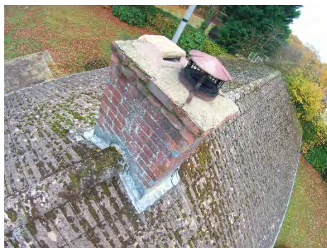
Spalled bricks, capped flue and poor flaunching
