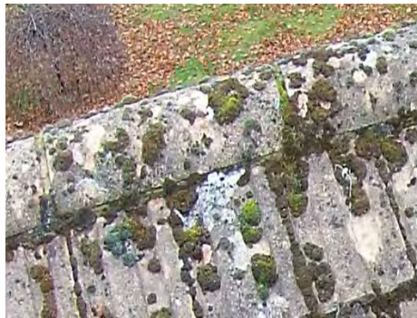
Mortar to the ridge and hip tiles is loose and cracking
