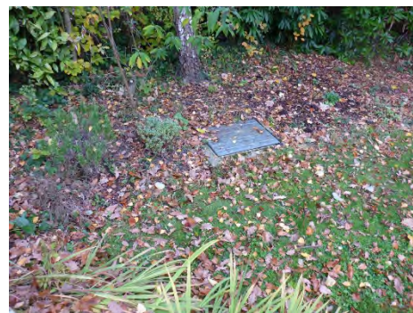
Cesspit inspection chamber cover to the rear
