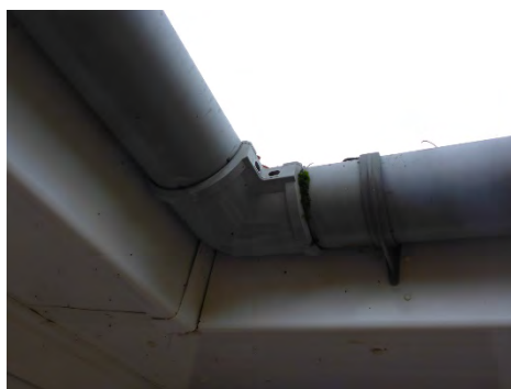
Leaky gutter joint to the front
