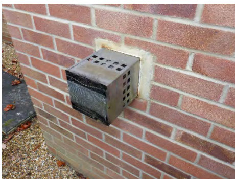
Boiler flue
