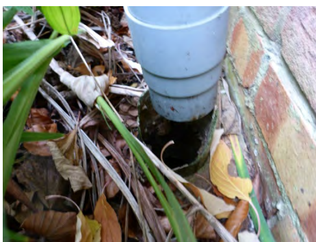
Broken rainwater connection
