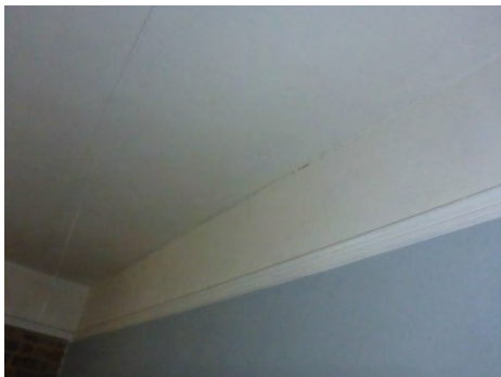
Ceiling line cracks
