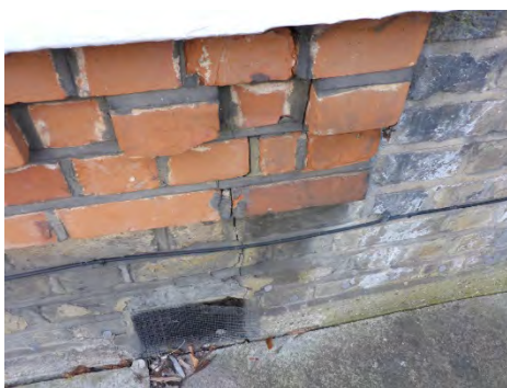
Cracks to the brickwork around the front bay window
