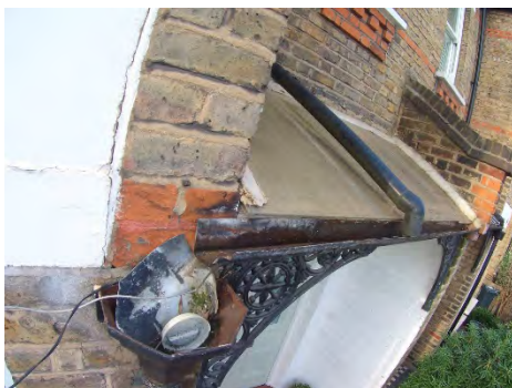
Porch guttering is blocked and in a poor state of repair
