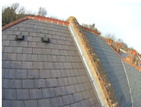
Lead flashing are longer than 1.5m
