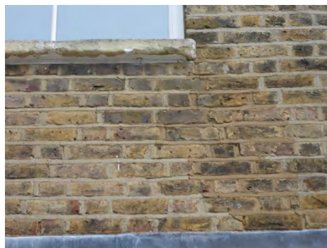
Cracks above conservatory
