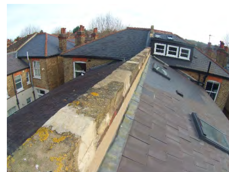
Rear parapet wall in a poor condition
