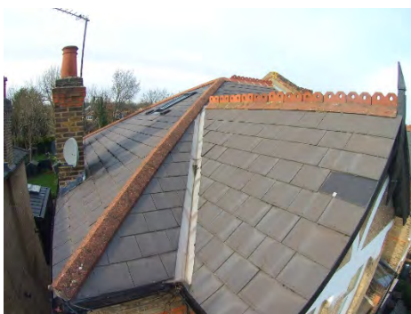
Poorly repaired slate to the front
