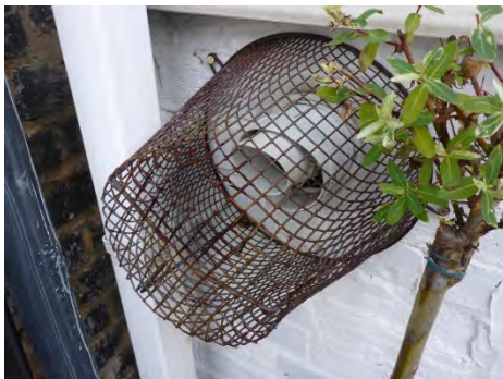
Fan assisted flue
