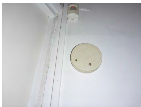
Battery powered smoke detection
