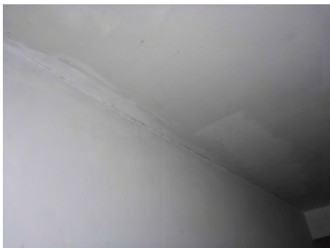
Ceiling line cracks
