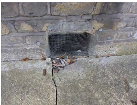
Front air bricks are damaged
