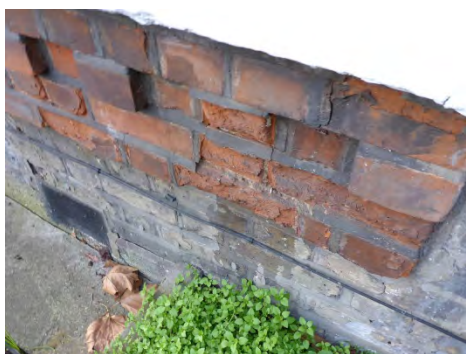
Spalled bricks to the front bay window
