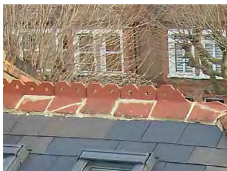
Broken ridge tiles to the main roof
