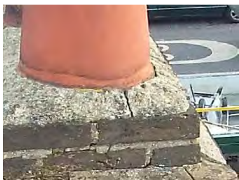
Cracked and defective flaunching
