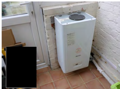
Wall mounted boiler
