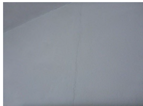
Wall cracks
