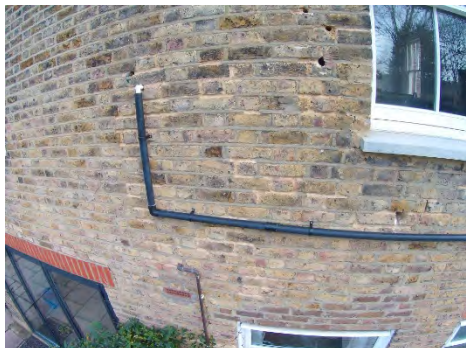
Loose and defective pointing to the rear walls
