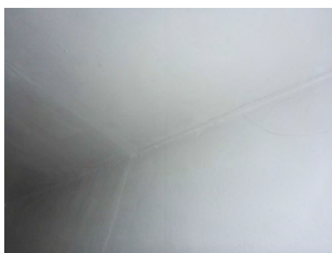
Ceiling line cracks
