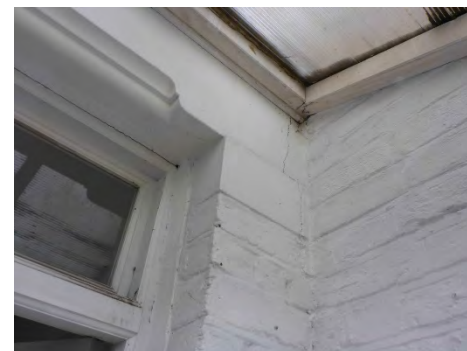
Cracks inside the front porch
