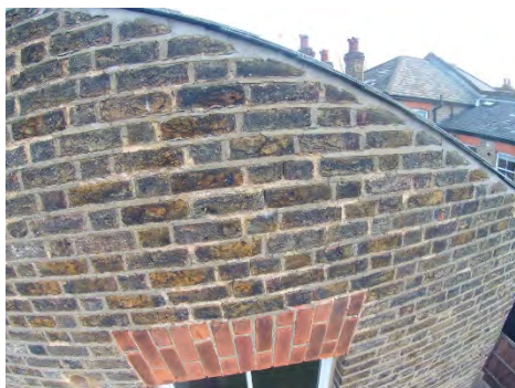
Cracks above rear off shoot window
