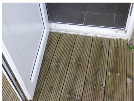
Rear decking is finished too high against the building
