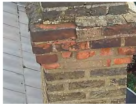
Spalled bricks and loose pointing
