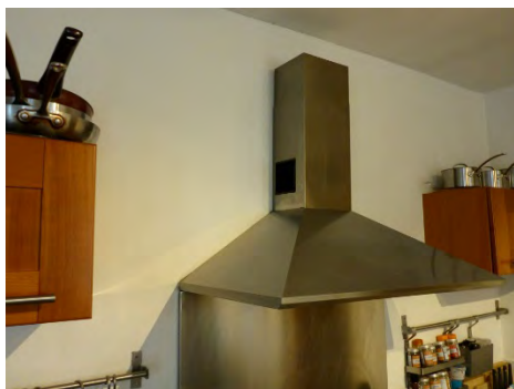
Extractor is not externally ducted
