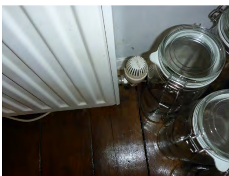
TRV's fitted to one radiator
