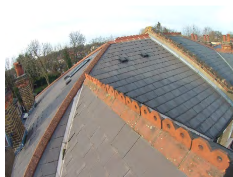
Loose and defective mortar to the ridge/hip tiles
