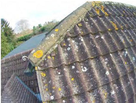
Loose and defective mortar to the ridge and hip tiles, valley tiling and verge tiling
