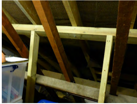
Additional supports installed to front and rear slopes
