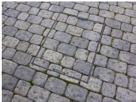
Inspection chambers to the right side
