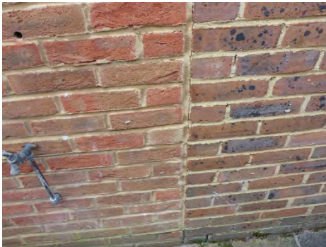
Vertical cracking at the junction between the original and extended walls
