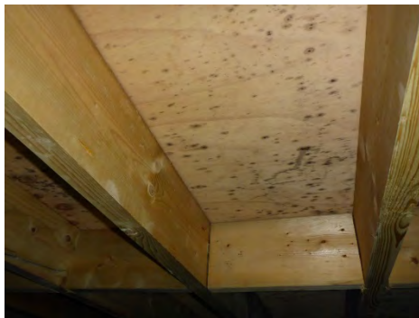
Mildew and mould growth to the underside of the flat roof decking
