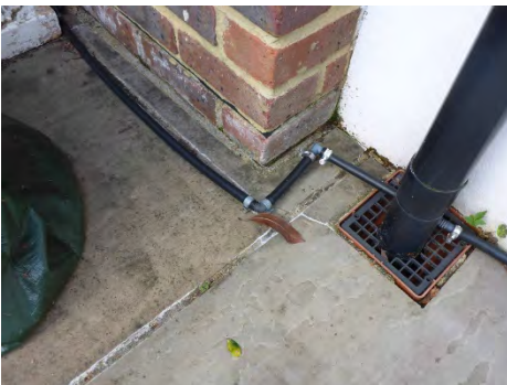
Open rainwater hoppers
