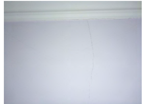
Wall cracks
