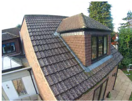
Rear roof slopes
