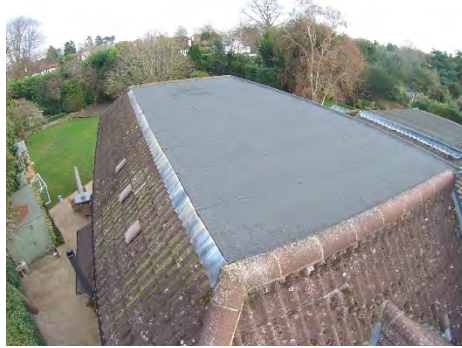
Side flat roof
