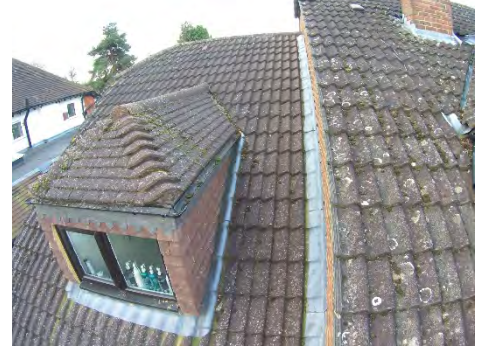
Rear roof slopes
