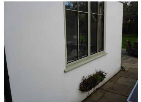
Aluminium windows and doors to the rear
