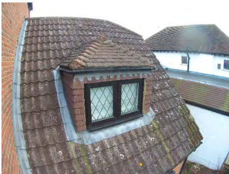
PVCu windows to the front sides and rear
