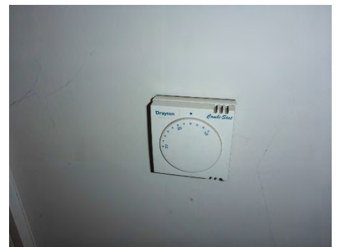
Thermostatic control
