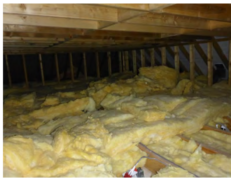
Additional supports installed to front and rear slopes
