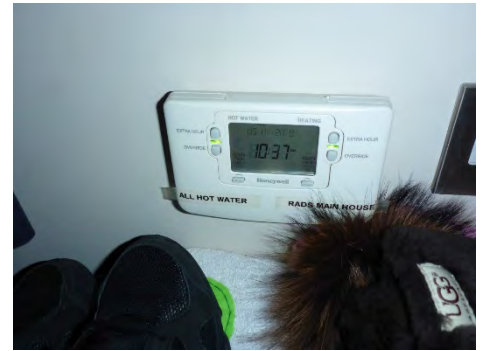
Boiler programmer
