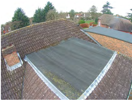
Rear dormer flat roof
