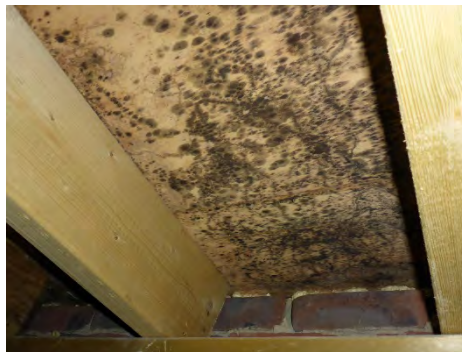
Mildew and mould growth to the underside of the flat roof decking
