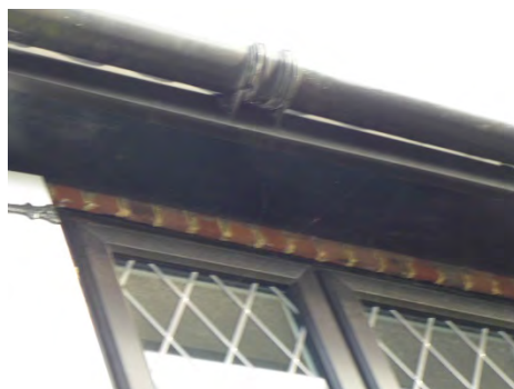
PVCu soffit and fascia boards
