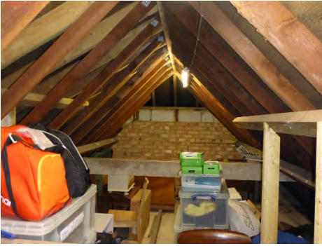
Main roof is well braced and supported
