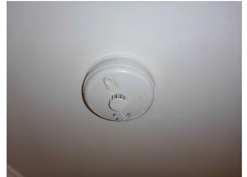
Mains powered smoke & heat detection
