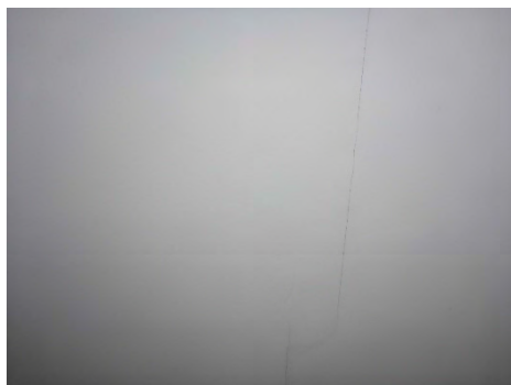
Ceiling cracks
