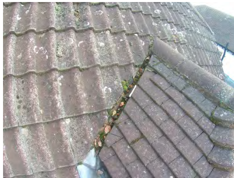
Loose and defective mortar to the ridge and hip tiles, valley tiling and verge tiling
