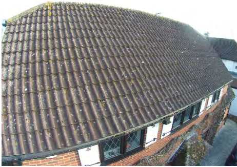
Front roof slope
