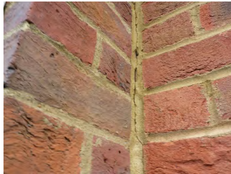
Vertical cracking at the junction between the original and extended walls
